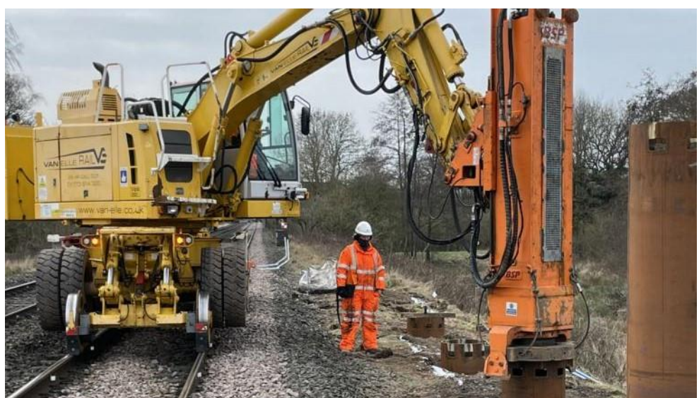
Figure 5: Rail work in progress
