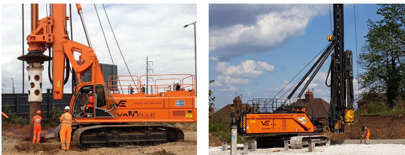
Figure 19: Rotary bored (LHS) and driven piling (RHS)
