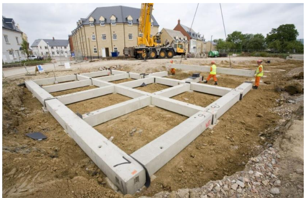
Figure 20: Smartfoot foundations in place on housing development
